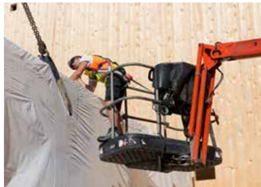
As a rule, components for long spans need to be assembled at greater working heights. For making your employees' on-site work as safe as possible, you need to provide suitable fall protection equipment.
