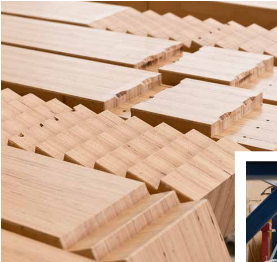
Trimming BauBuche beams and cutting a multiple step joint to take up compressive loads.
