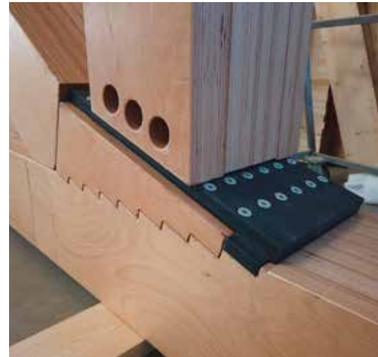
Example of an extended multiple step joint
